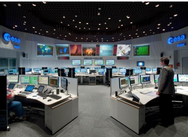
Main Control Room
